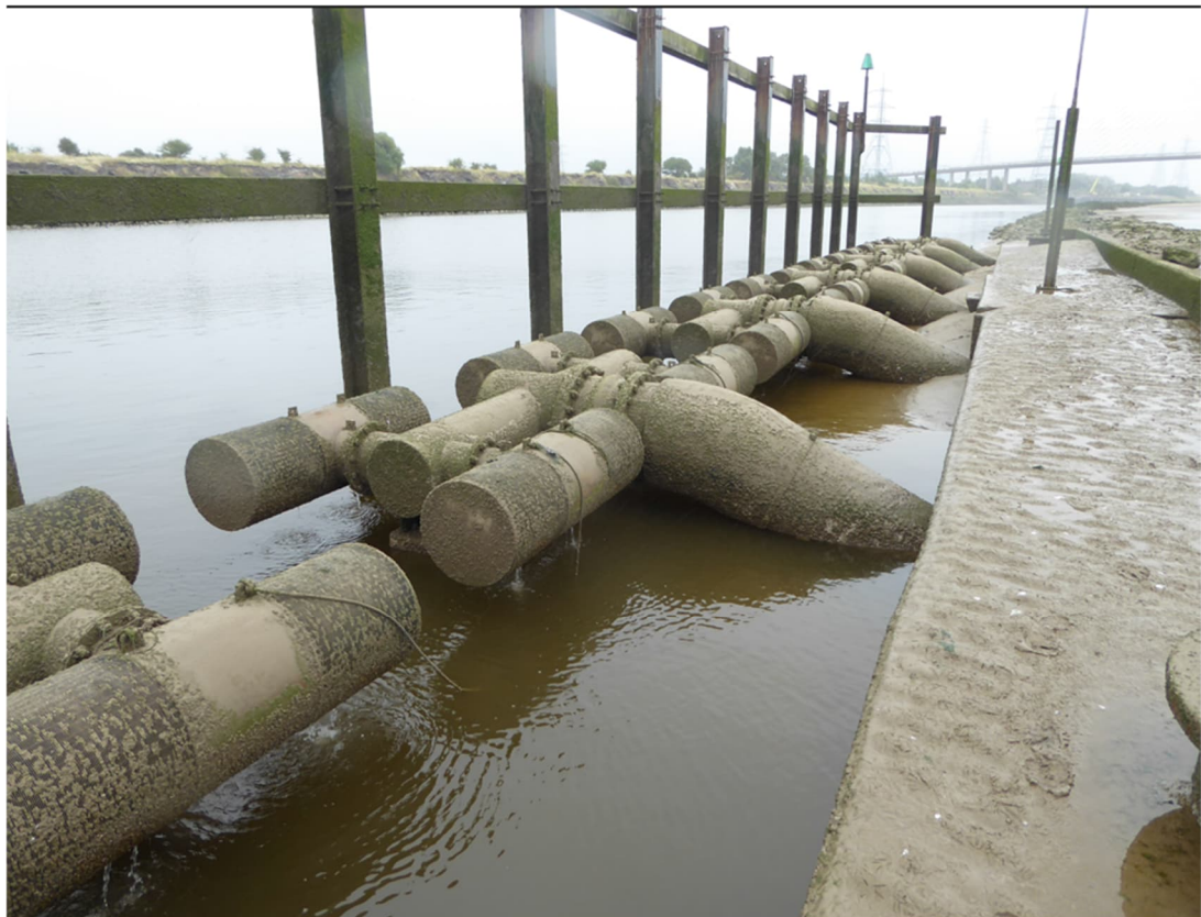
Plate 1: Photograph of existing intake eel screens, intake manifold and steelwork protection
